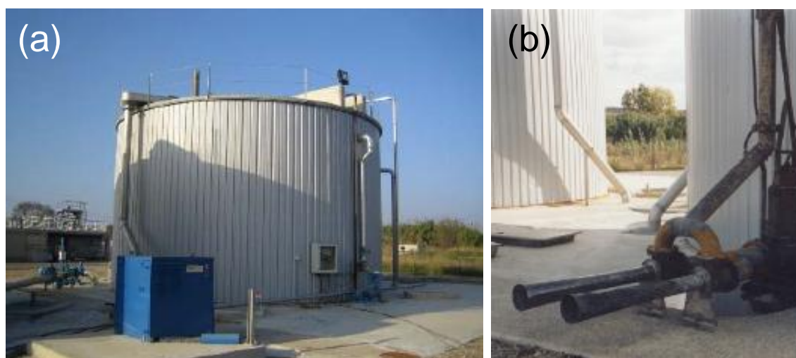
Figure 5.1: Photograph of (a) single-stage ATAD system CS1, and (b) Venturi jet aerator. Adapted from Gomez et al. (2007) and Gomez (2007).
