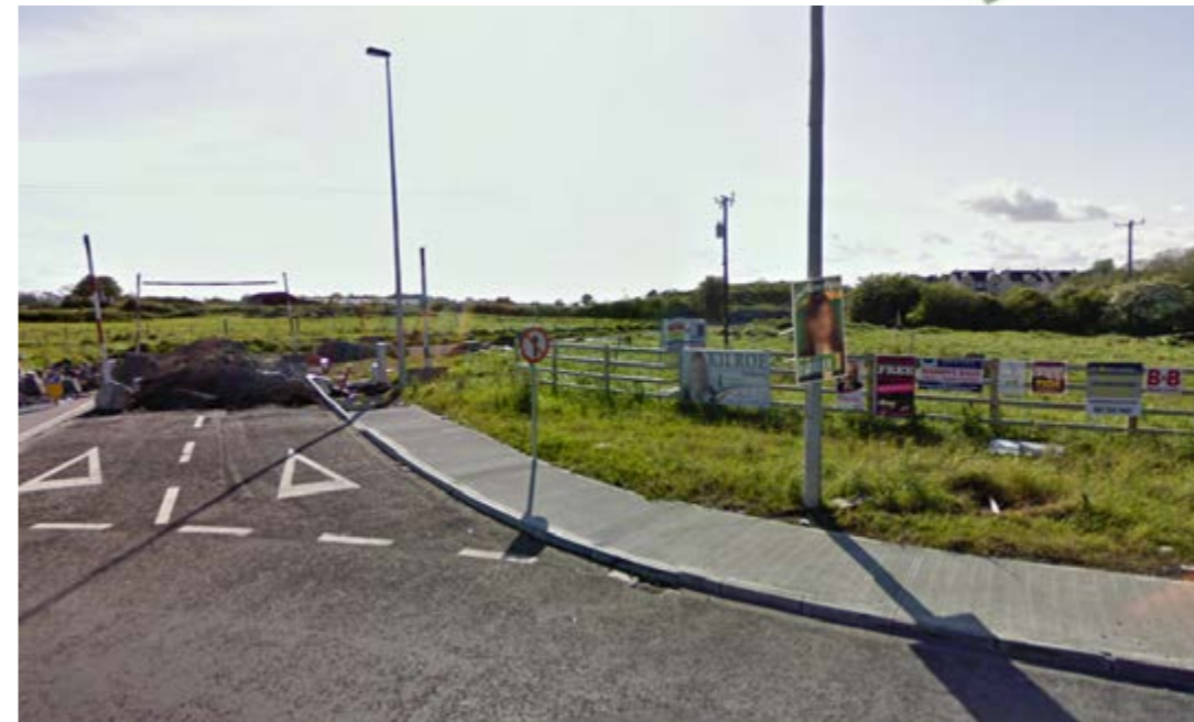
Fig 5 halted development at roundabout existing Oranmore along the N17 in the Clarinbridge direction.
