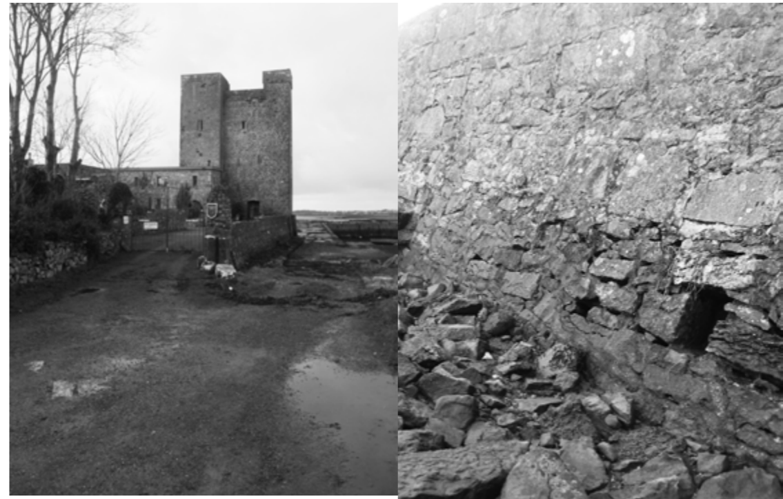
Fig 30 & Figure 31 (above) Current view approaching Oranmore Castle & wall detail
